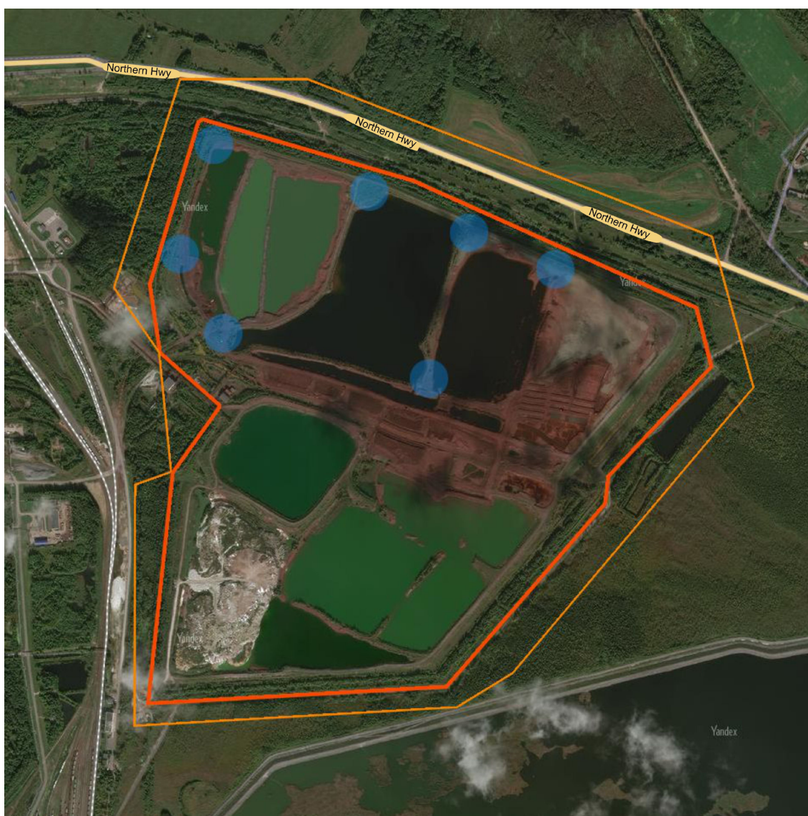
Fig. 1. Sludge reservoir of pyrite cinders in the vicinity of Cherepovets. The orange line shows the border of the sludge reservoir, the yellow line shows the border of the adjacent zone, the studied areas are marked with blue filling.
